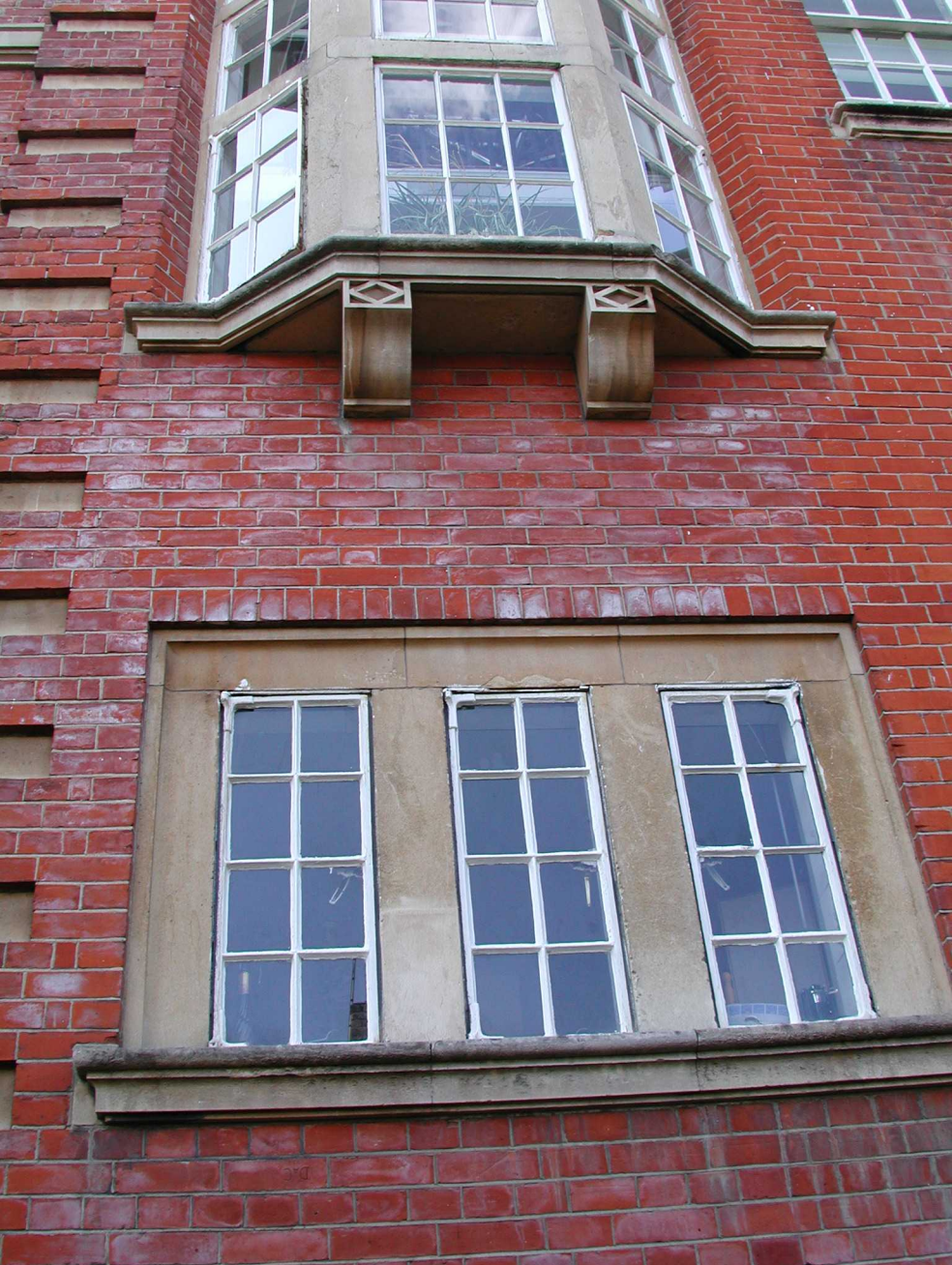
This was called the Prefects' Parlour - a window on the stairs to the Boiler Room
